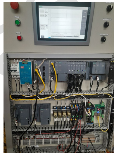
Fig. 9. The S7 1500 PLC turbine control system
